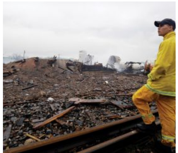
Associated Press/Photo by LM Otero DEVASTATION: A firefighter surveys the remain the fertilizer plant.
